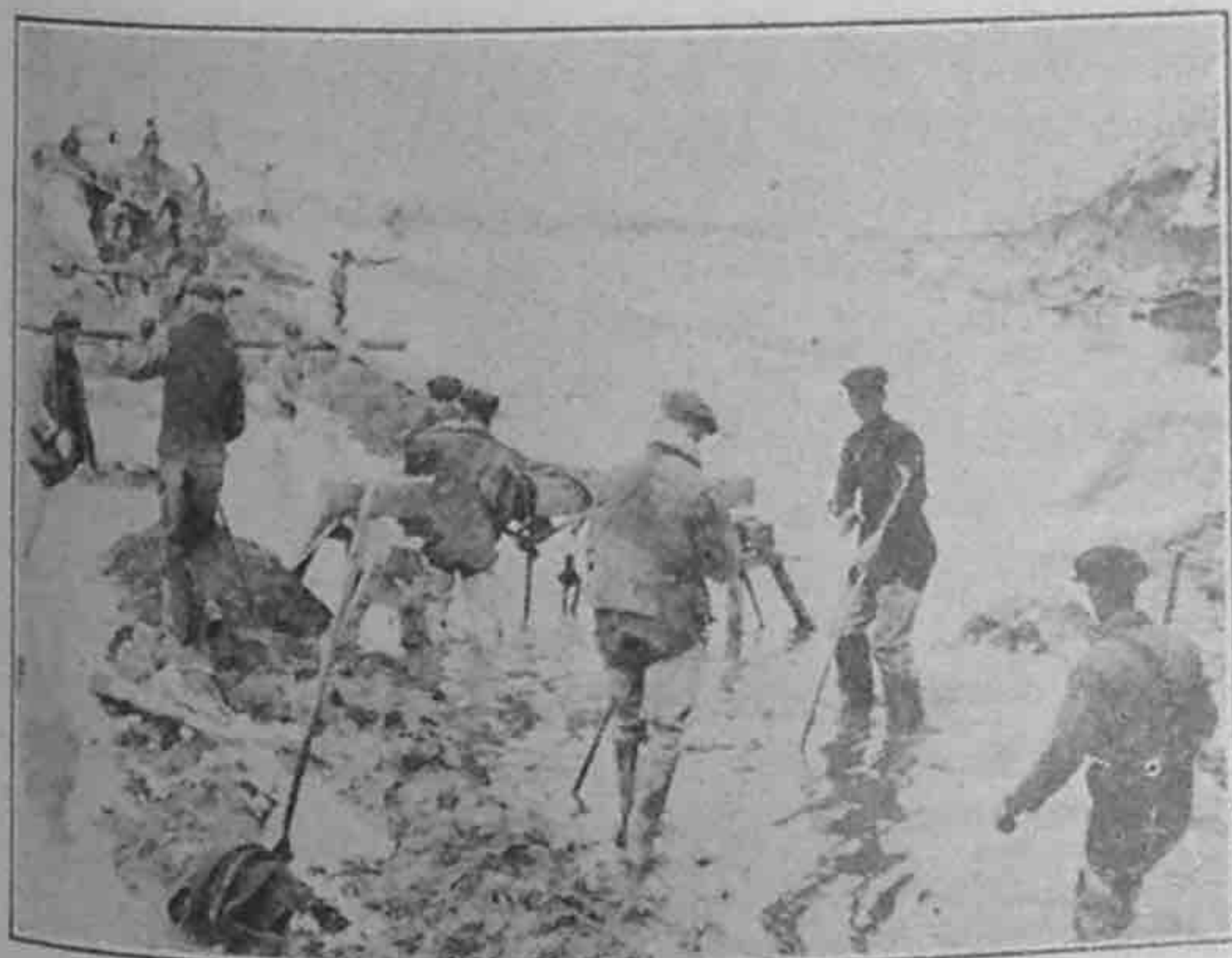
Pipeline Laying in Wyoming
