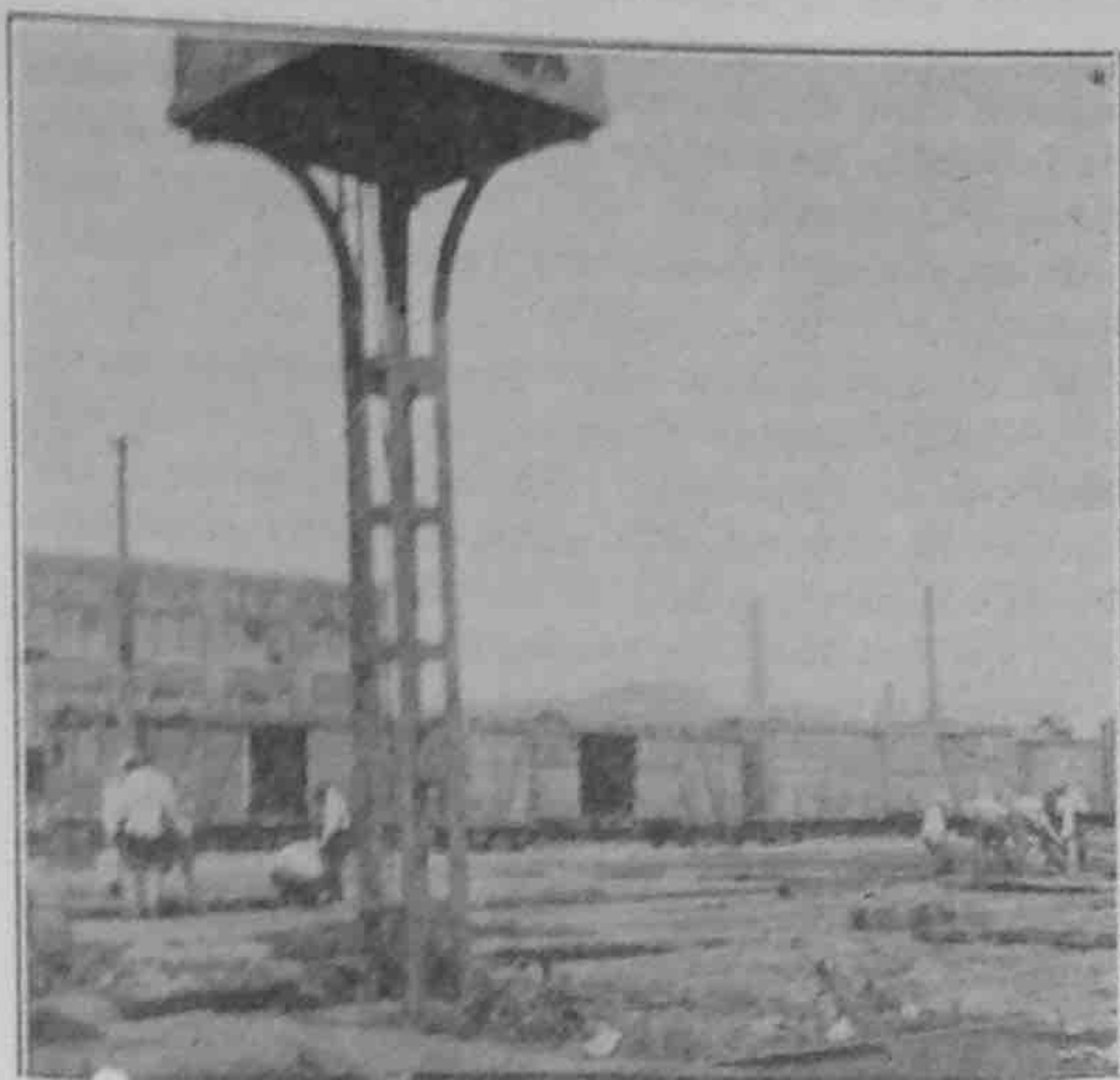
Repairing a Crossing
